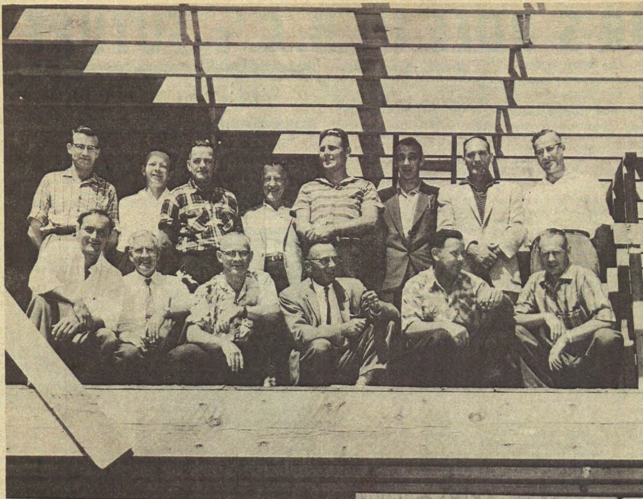
The Provincial Executive of Local 180 inspect progress on new headquarters. Situated on Broadway in the 300 block, the new two storey building should be available for occupancy in October. Executive members are, seated left to right, Tony Burrell, 2nd Vice-President, North Burnaby; Alex Paterson, Financial Secretary, V.G.H.; John Fleming, Provincial President, Royal Columbian; W. M. "Bill" Black, Secretary-Business Manager; W. D. Black, Trustee, Royal Columbian; Albert Tetz, Okanagan District Council Representative. Standing left to right, Jim Spracklin, 3rd Vice-President, V.G.H.; W. "Wally" Lake, Maple Ridge; Phil Sevin, Trustee, V.G.H.; Hugh Duff, Trustee, V.G.H.; Gerald Larson, Lower Mainland District Representative; Joe Gallagher, 1st Vice-President, Powell River; Harold Cole, Kootenay District Council; R. Louis Woodthorpe, Vancouver Island District Council Representative.
