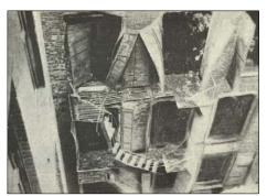
Many of the casualties could have been avoided. There was no fire alarm. Emergency doors were locked by the employer to prevent theft. A sprinkler system wasn't installed. Stairwells were only two-feet wide, making it challenging for workers to escape. The fire department's ladders only extended to the sixth floor – 30 feet below the terrified workers awaiting rescue at the smoke-billowing windows.
